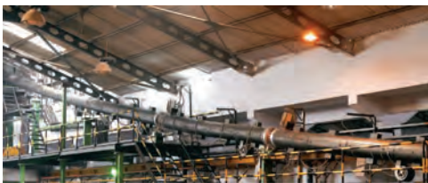
Figure 1 : 6 Nos. CCV (DRY CURE) LINES
